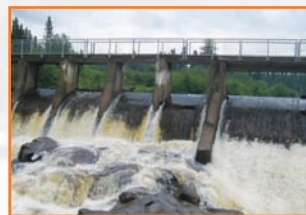
Dam Walls • Saguenay
