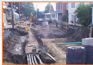
Upgrading water supply and sewer • Boischatel
